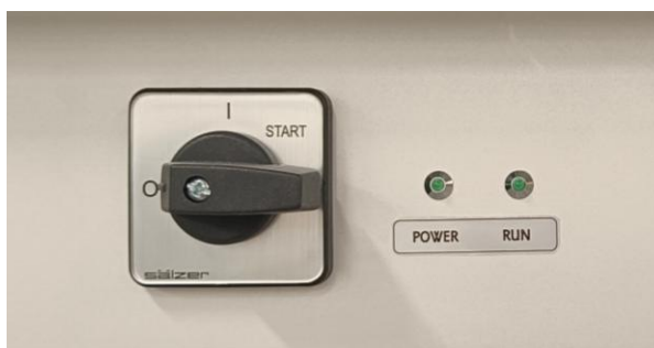
Fig. 15-1 System switch located in the electronic rack with Power and Run LEDs.
