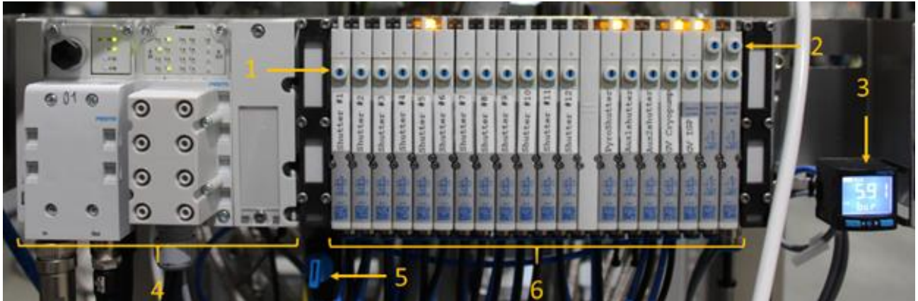
Fig. 9-2 Example FESTO controller for pneumatic valves: 1. Manual override actuator for individual pneumatic lines (single solenoid coil), 2. Manual override actuator (dual solenoid coils), 3. Air flow sensor (if applicable), 4. Digital periphery of FESTO controller with communication Profibus® interface, 5. Compressed air shut-off valve, 6. Pneumatic section of FESTO controller.
