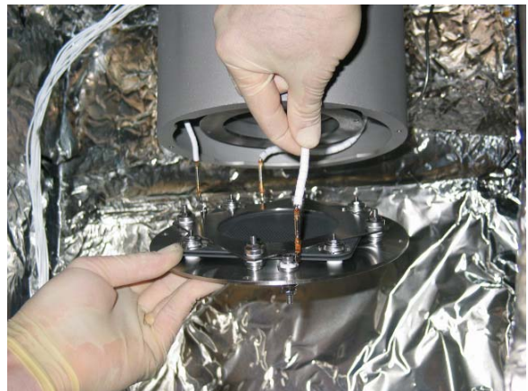
Picture 4.26. Electrical lead attachment.
