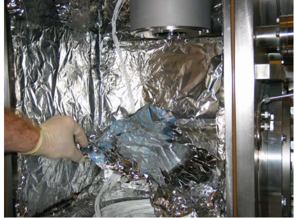
Picture 4.32. Protection of electrical leads.
